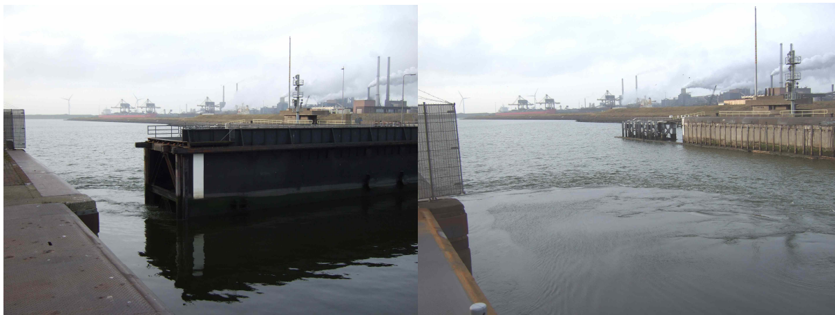
Figure 2: Fresh water tongue spreading over saltwater after opening the lock gate at IJmuiden, The Netherlands
