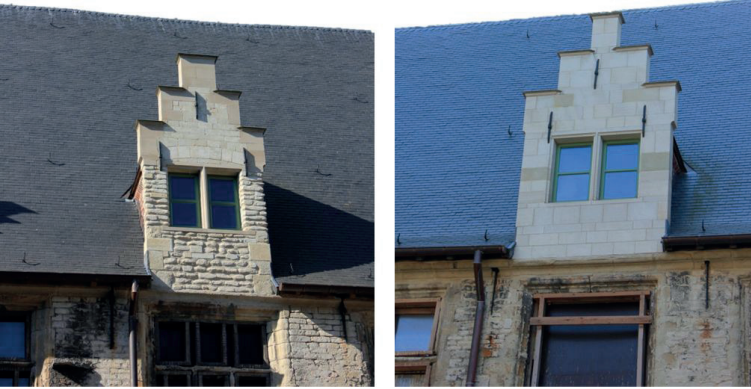
Figure 8.2: Wall dormers in the Caermers monastery in Ghent. Left: the bottom of the water dormer is retained in Brussels stone (masonry) and Lede stone (corners), whilst the top of the wall dormer is replaced with Gobertange stone (masonry) and San Louis (corners). Right: wall dormer originally in Lede stone which is now completely replaced by San Louis.
