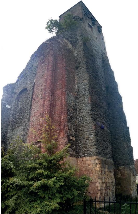
Figure 9.1: Tower ruin in Dudzele as seen from the northwest. The lower façade is mainly built with buff-coloured limestone, the upper masonry with Fieldstone and parts in brick.
