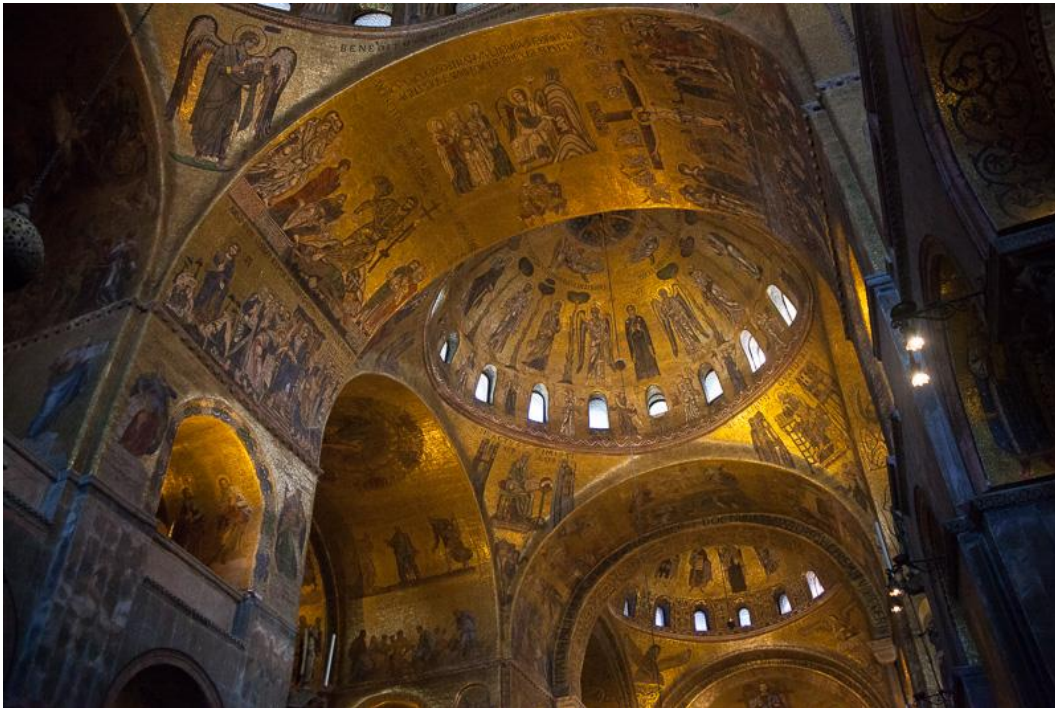
Fig. 86. Decorated spandrels in the Basilica San Marco, Venice. The architectural combination of adjoining arches covered by a dome creates tapering triangular spaces, which have been co-opted for decorative purposes.
