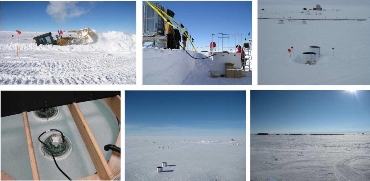
Figure 2.7: The deployment of IceTop tanks in 6 steps: Top left: The bulldozer is digging a trench for placing an IceTop station, Top center: Two tanks are placed in a trench, with their top level with the snow surface and filled with filtered water, Top right: Sunshade are installed and the water in the tanks is freezing. Bottom left: View of 2 DOMs in a tank during freezing. A thin layer of drifted snow is visible (before it was removed) and the pipe used to fill the tanks is also visible. The tanks freeze with the lid open to limit insulation from the cold. Bottom center: Trenches are backfilled and several stations are still freezing. Bottom right: On the left the lids of two tanks are visible. The sunshades have been removed, the tanks filled with perlite and the lids closed.
