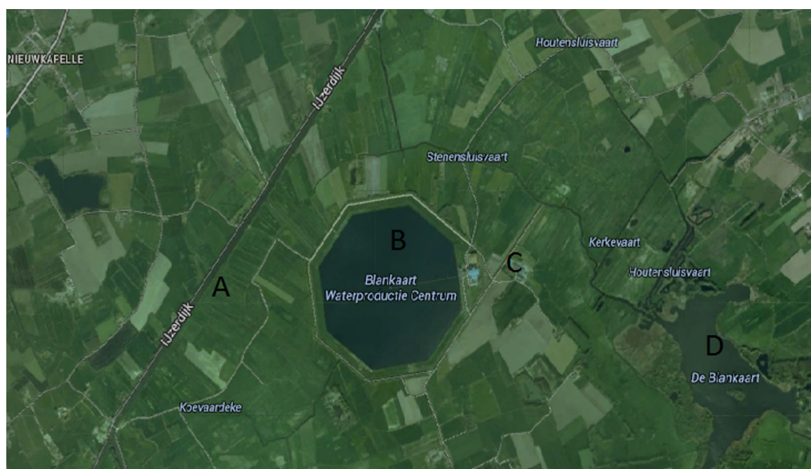
Figure 2.1 Picture of the Blankaart catchment site. A Yzer river, B water storage basin, C water supply channel from the Yzer river and D the Blankaart nature reserve.
