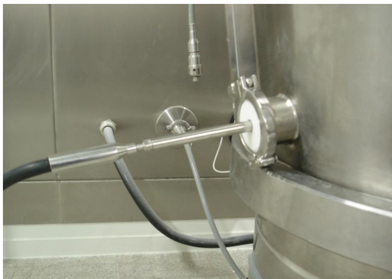
Figure 8.1. NIR fiber optic contact probe mounted in cell 5 of the dryer by means of an in-house made accessory.
