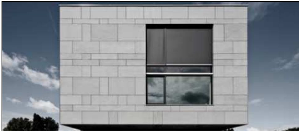
Figure 7.4.: Example of a autoclaved FC façade product (source: www. eternit.be [cited 2014 Apr 30])
