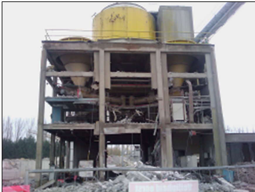
Figure 10.8.: The old concrete plant of Inter Beton Sint-Pieters-Leeuw (Belgium)
