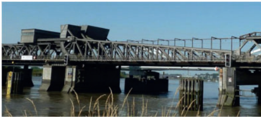
Figure 3. Movable part of the Temse bridge.
