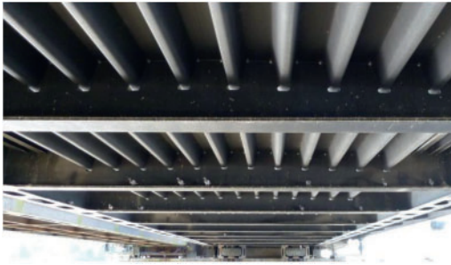
Figure 4. Orthotropic deck plate of the Temse bridge.
