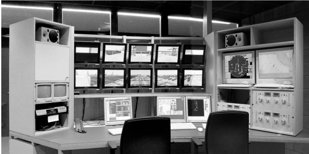
Figure 1.11. Flanders Hydraulics Research: operator's room of SIM360+.
