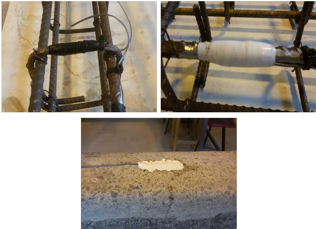
Figure 3.15: Concrete and steel strain gauges after protection.
