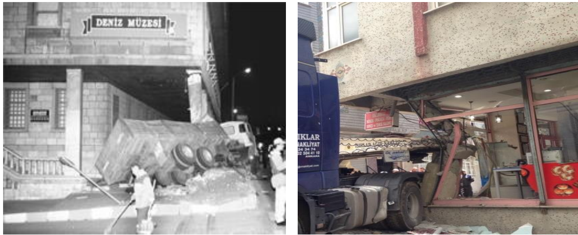
Figure 1.1: Examples of damage caused by vehicle collision (Gomez, 2014; Buth et al., 2010).
