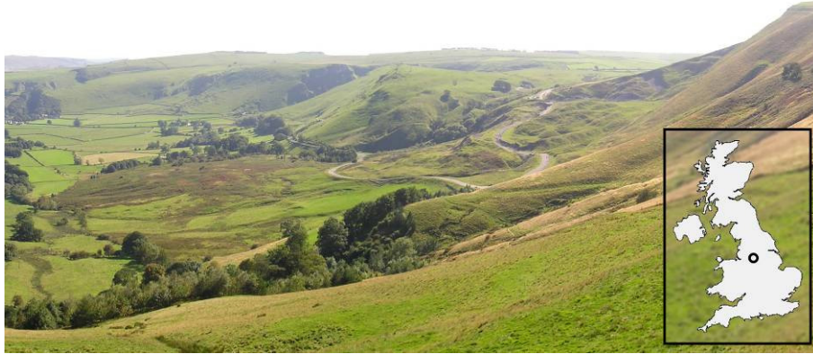
Fig. 5. The Mam Tor landslide: head scarp on the right, debris slide on the left side, and the abandoned road crossing the central area. Inset: location of Mam Tor.
