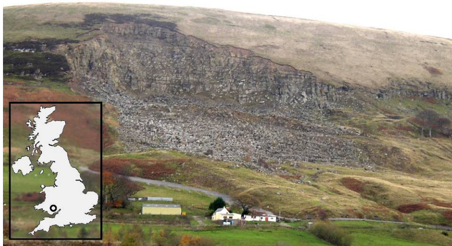
Fig. 13. The East Pentwyn landslide: head scar visible at the back, the boulder field in the central part and the two vegetated debris slide lobes below. In the forefront is East Pentwyn farm. Inset: location of East Pentwyn.
