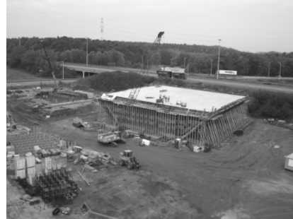
Fig. 3: Construction site near E313 – Lummen - source: Jan De Nul NV, 2008
