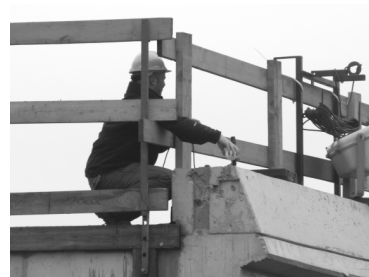
Fig. 8: Attachment of spherical target to upper side bridge element
