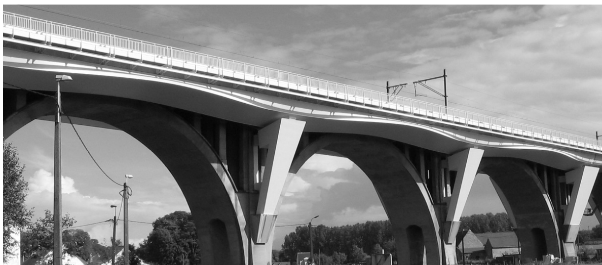
Fig. 1. Front view of the new steel super structure.
