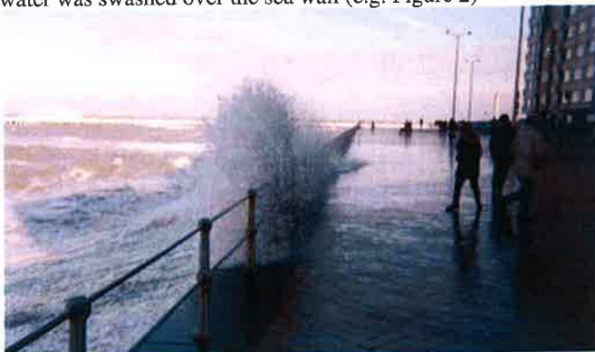
Figure 2: Overtopping event during a storm with small return period before 2004
