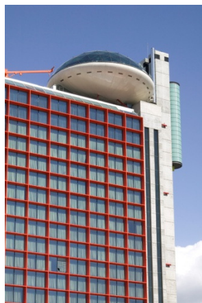
Fig. 5 EVO restaurant on top of the hotel (Photo: Bellapart S.A.U.)
