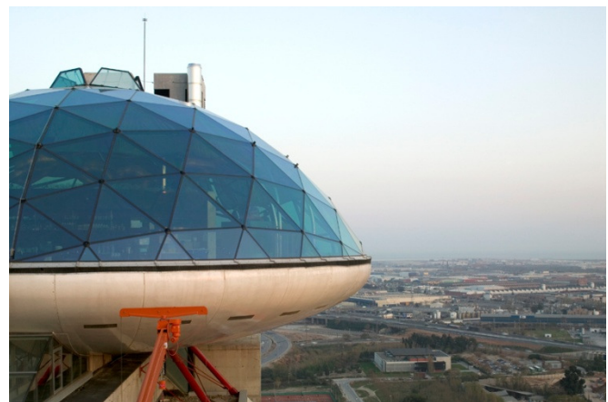
Fig. 6 Glazed dome of the restaurant on top of Hotel Hesperia (Photo: Bellapart S.A.U.)
