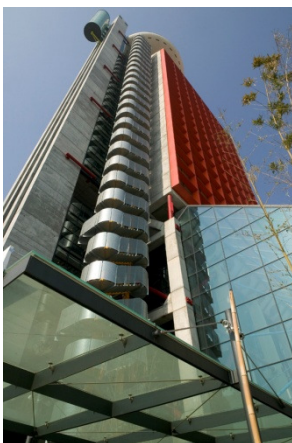
Fig. 4 Hotel Hesperia in Barcelona, upwards view (Photo: Bellapart S.A.U.)
