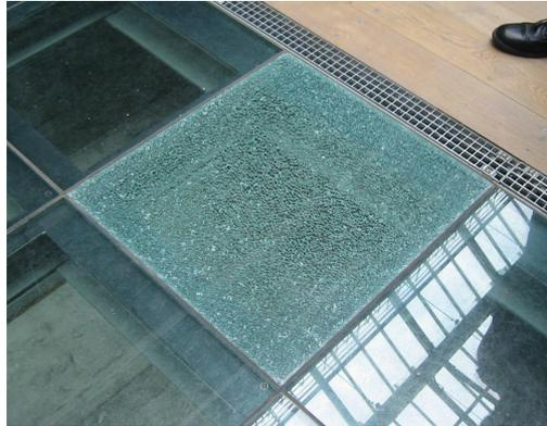
Figure 1: Practical example of post-breakage stadium : a floor element in laminated glass with the upper ply broken is expected to show residual resistance
