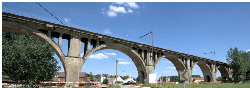
Figure 1: Front view of the historic Pede viaduct.
