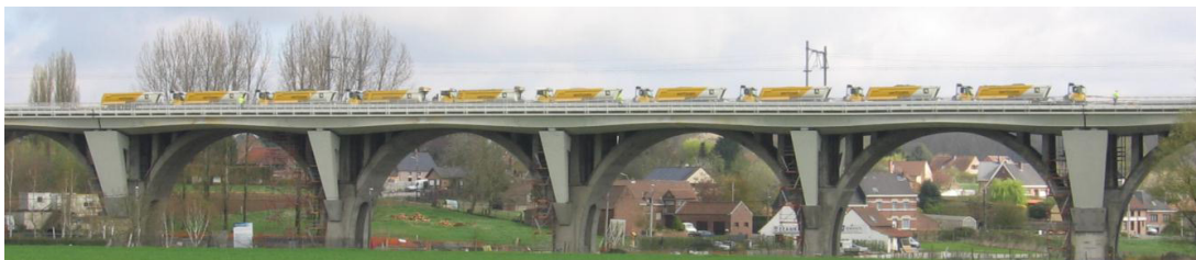
Figure 18: Load test of a continuous 4-span deck using heavy lorries.
