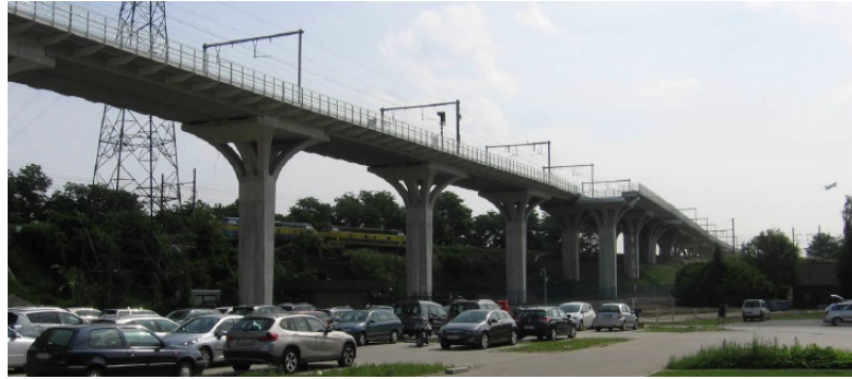
Figure 2: Part of the Iris viaduct in Haren, Brussels.
