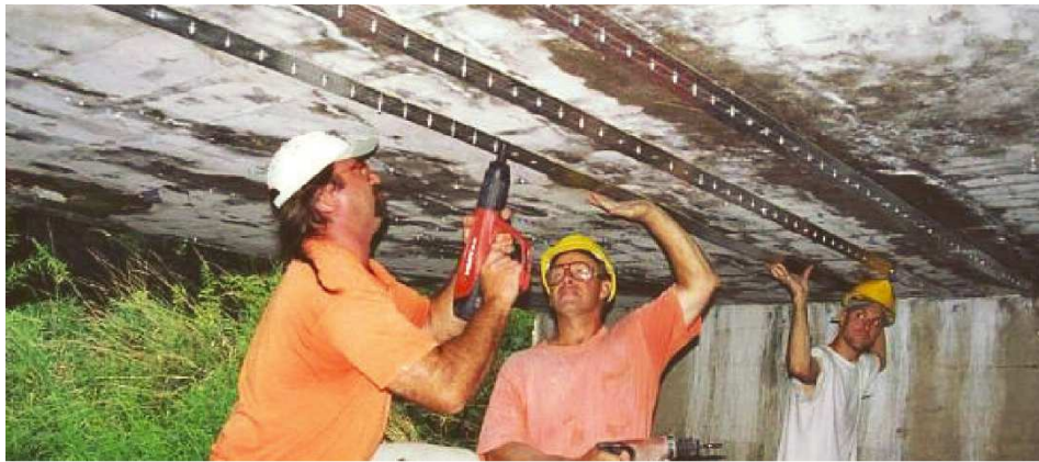
Figure 2.22: Installing MF-FRP strips on the Edgerton Bridge [62]
