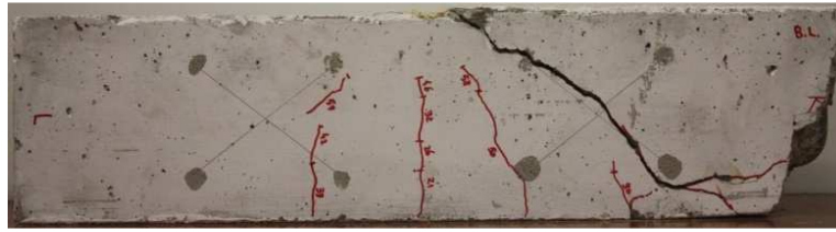
Figure 4.36: Crack pattern of beam CB at the end of the test
