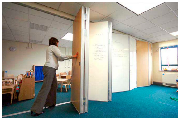
Figure 2. Example of removable partition wall (Dividers, 2014).
