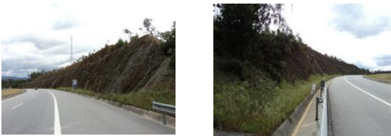
Figure 1. General view of the selected slope.
