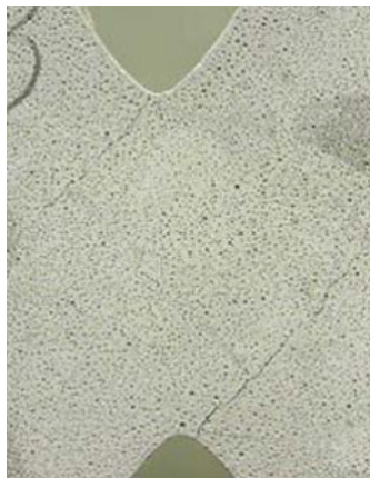
(a) final crack pattern of PCM (Shang and Zijl 2007)
