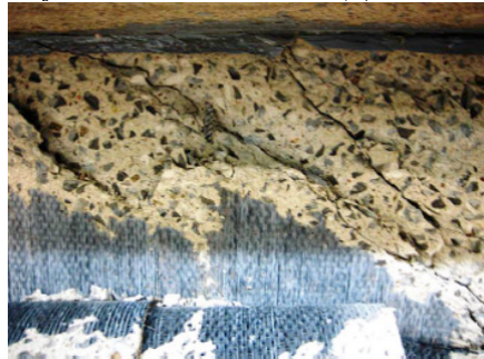
(c) beam with shear reinforcement and reinforced with EB FRC sheet
