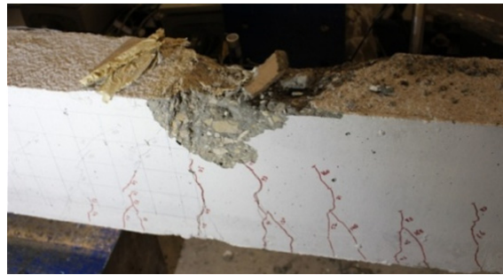
Figure 3-14: Crack patterns and failure modes of the 7S-R-I beam
