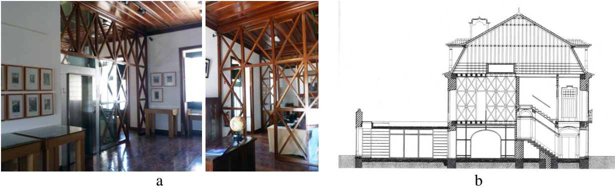
Fig. 7. (a) Aesthetic reconstruction of frontal walls in the south riverfront ‘tower’; (b) Cross section of the rehabilitation project of the South riverfront ‘tower’ [17].
