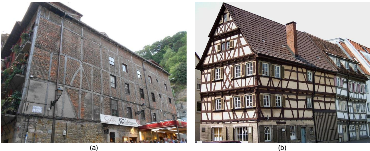
Fig. 1 Examples of timber frame buildings: (a) historic buildings in calle 31 de Agosto, San Sebastián, Spain; (b) typical timber frame buildings in Sindelfinge, Baden-Württemberg, Germany
