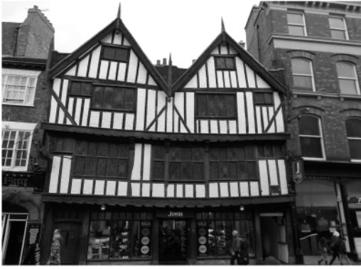
Figure 1. A XV century timber frame house in York, England (credits: E. Poletti).
