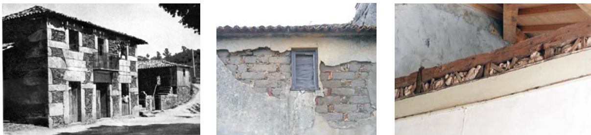
Figure 1: Examples of Portuguese vernacular architecture and traditional materials commonly applied: (from left to right) stone [6], earth [9] and timber
