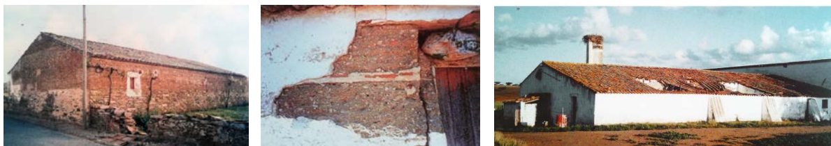
Figure 3: (left) Stone base course [20]; (middle) brick masonry horizontal course within rammed earth walls [20]; chimney [20]
