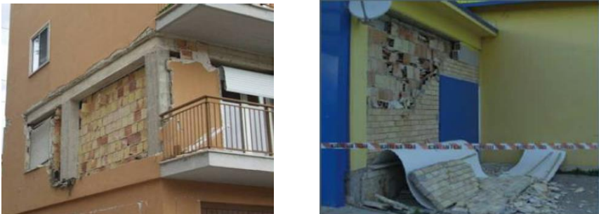
Figure 3 Detachment of the leaves in multi leaf walls (Braga, Manfredi et al. 2011)
