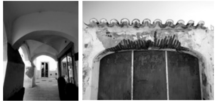
Figure 5. a) Arcades and vaults system in the historical centre of Évora . b) Flat arch or Jack Arch, Castro Marim (Credits: CI-ESG).
