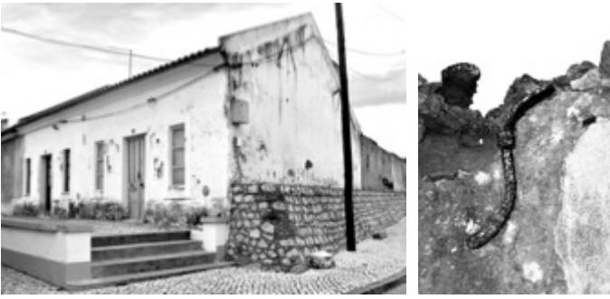
Figure 4. a) House in Benavente , with tie rods and plinth as reinforcements. b) Metallic anchoring device (cat), Melides . (Credits: CI-ESG).
