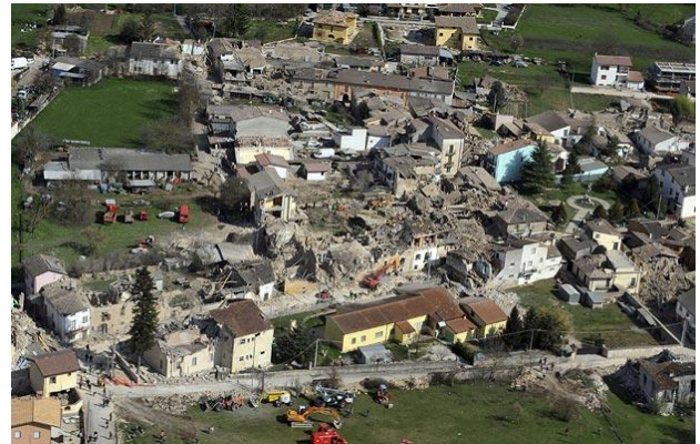
Figure 4 – Village affected by the L'Áquila earthquake
