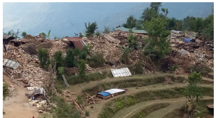
Figure 9 – Collapsed houses of an entire community near Barpak during the Gorkha earthquake, 2015 ©DipendraGautam 2015
