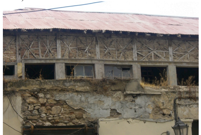
Figure 2 – Timber elements within walls in Greece
