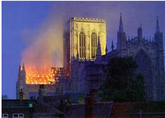
Figure 2-25. In 1984 a great fire, believed to have been caused by a lighting strike, destroyed the timber roof of the south transept of York Minster. Additional damage was caused by the vast quantities of water used to put out the fire. ("An Introduction to the History of York" 2014)
