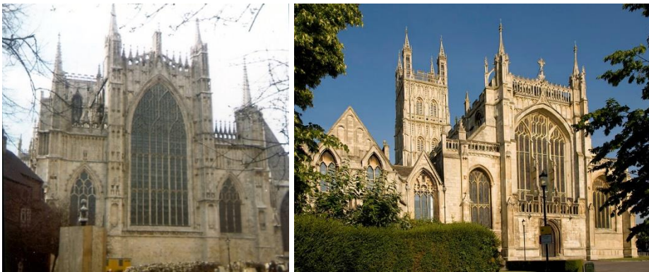
Figure 2-4. (Left) York Minster Cathedral, England, York (1338-1408). Equilateral arches at the east front ("York Minster" 2014). (Right) Gloucester Cathedral, England (1089–1499). Depressed arches at the east front ("Gloucester Cathedral" 2014).
