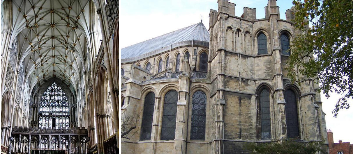
Figure 2-16. (Left) East end in York Minster Cathedral, showing the typical square configuration ("York Minster" 2014). (Right) East end of Canterbury Cathedral, having a semi-circular plan with three chapels ("Canterbury Cathedral" 2014).
