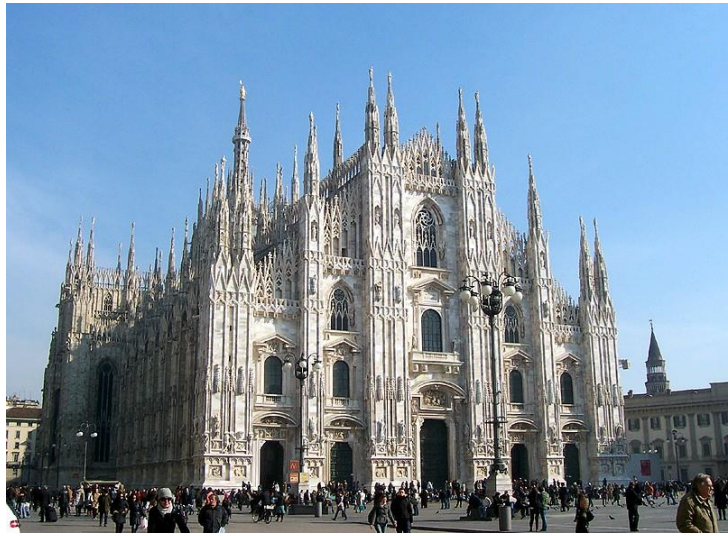
Figure 2-9. Milan Cathedral. Advanced use of pinnacles and spires in the vertical arrangement of piers, buttresses and roof gables ("Milan Cathedral" 2014).
