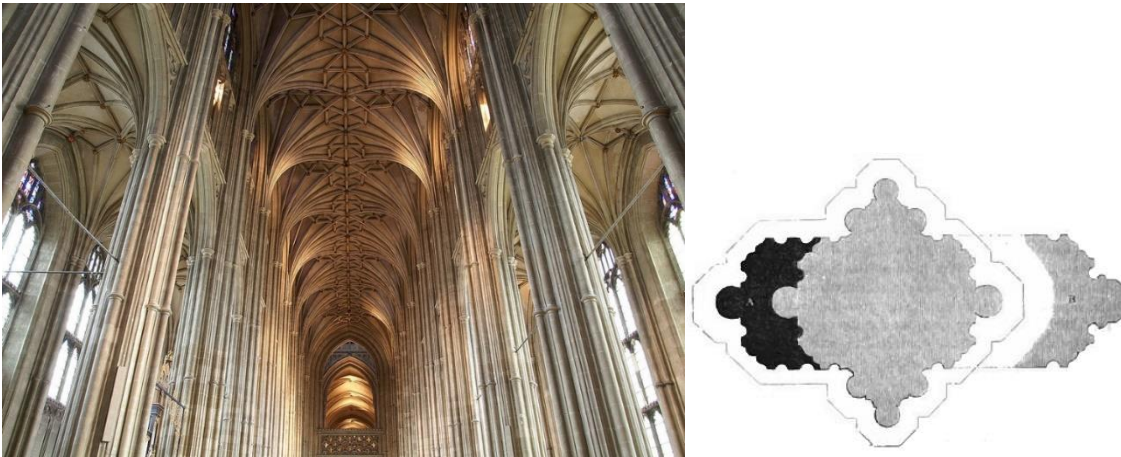
Figure 2-15. (Left) View of the central nave of the Canterbury Cathedral (1070-1834) in the UK. The pier molds are incorporated with the arch molds, resulting in a vertical continuity, thus creating a series of tree-like patterns ("Canterbury Cathedral" 2007). (Right) Pier section in the nave (center section), additional portion of the pier next to tower (left section) and arch mold (right section) (Willis 1845).
