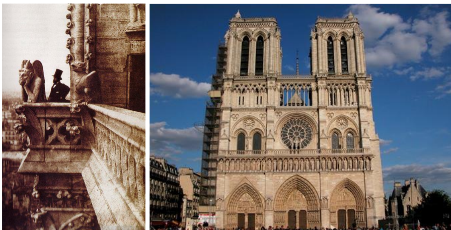
Figure 2-22. (Right) Notre Dame in Paris (1163-1345). From 1845-1870 the monument undertook a controversial restoration, resulting in many additions and reconstructions, such as the chimeras that were extracted from other Gothic buildings (Left) ("Notre Dame de Paris" 2014).
