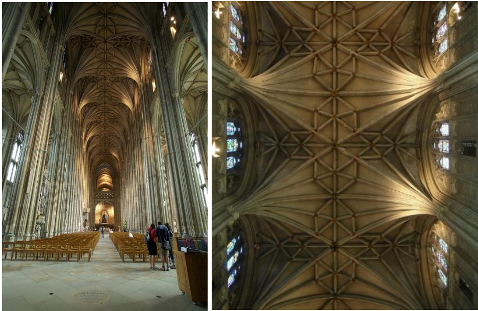
Figure 3-6. (Left) View of the nave of Canterbury Cathedral looking east. (Right) View of the Gothic lierne quadripartite cross vaults of the nave of Canterbury Cathedral (Photographic survey).
