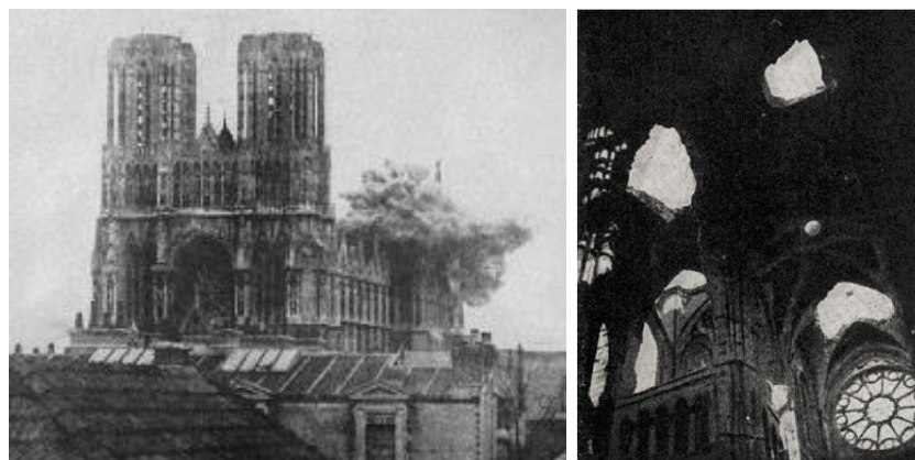
Figure 2-28. Reims Cathedral, Reims, France. (Left) Picture at the time of struck from German shellfire in September 1914. (Right) Inside view. Holes in the vault system from the bombarding (Theodossopoulos et al. 2008).
