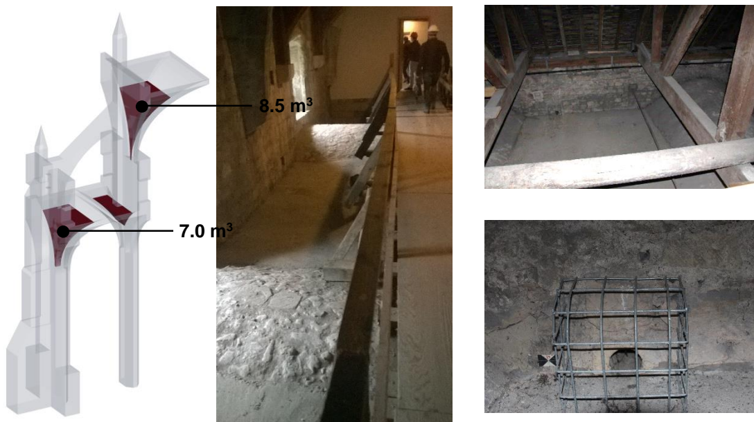
Figure 3-16. (Left) 3D representation of the south 3D CAD model of the critical nave section of Canterbury Cathedral, depicting the infill volumes. (Middle) Infill and cross vault system at south aisle roof void. (Right up) Infill and cross vault system at nave roof void. (Right down) Drilled hole in the exterior wall at the level of concrete layer infill, used for drainage (Photographic survey).
