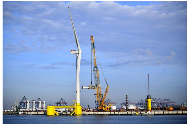
Fig. 4 Wind turbine assembly and integration at staging port
