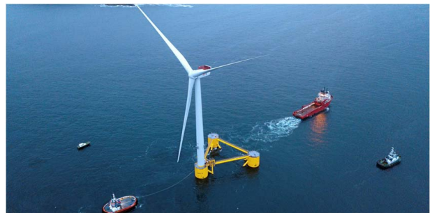
Fig. 5 Tow to installation site
