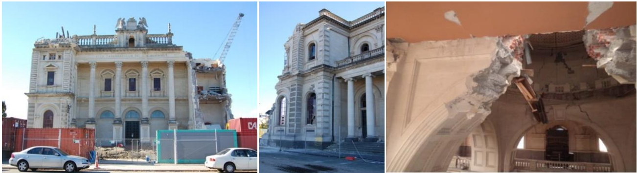
Figure 3. West façade of the Christchurch Catholic Basilica: damage at the two bell towers (left); Detail of the West wall collapse of the South bell tower (middle); Collapse occurred in the North arch of the sanctuary (right).
