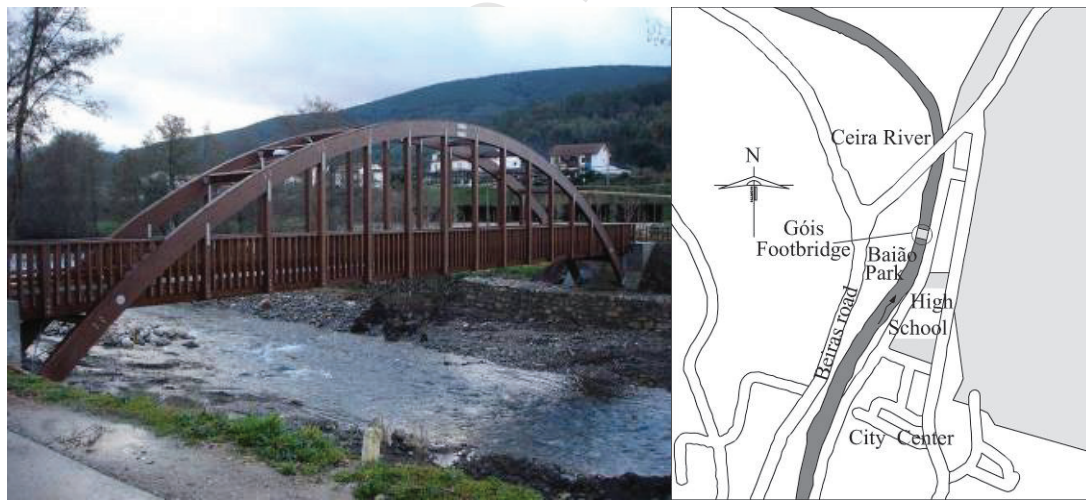
a) General view of the footbridge
