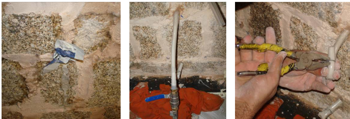
Figure 6: Walls grouting
