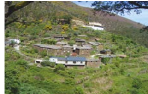
Figure 1 - Original Village of Rio de Frades
