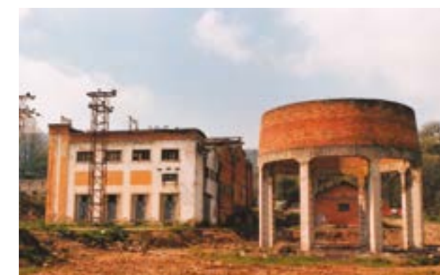
Figure 6 - Lena's power plant, abandoned since the early fifties. Ph. Victor Guerra, ab.1980
