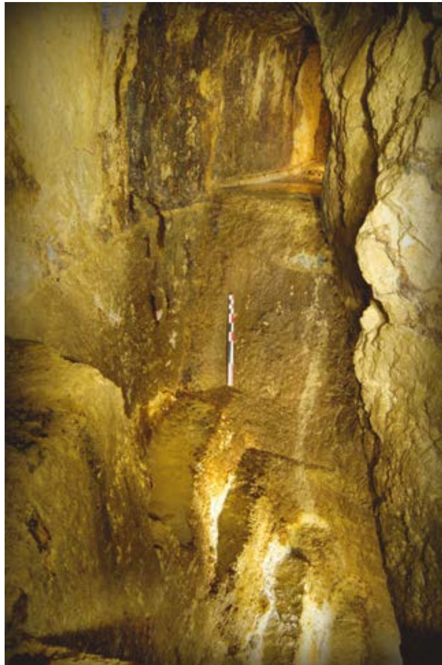
Figure 4 Large inclined shaft with steps dug at the bottom of Cârnic 3 network as an exploitation work and finally used as a collecting pit for water (Photo. J.-F. Peiré).
