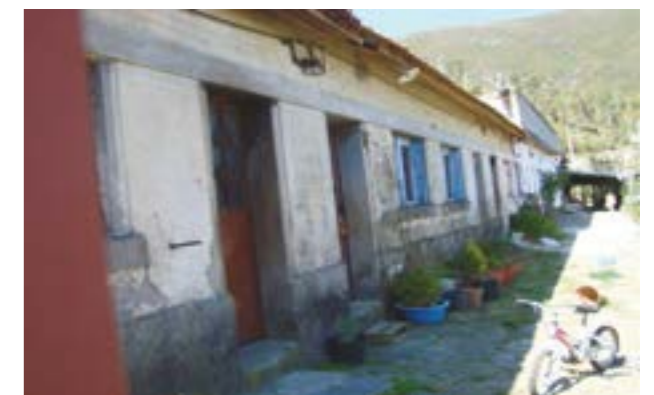
Figure 4 - Former miners's houses. Currently locals are living in them
