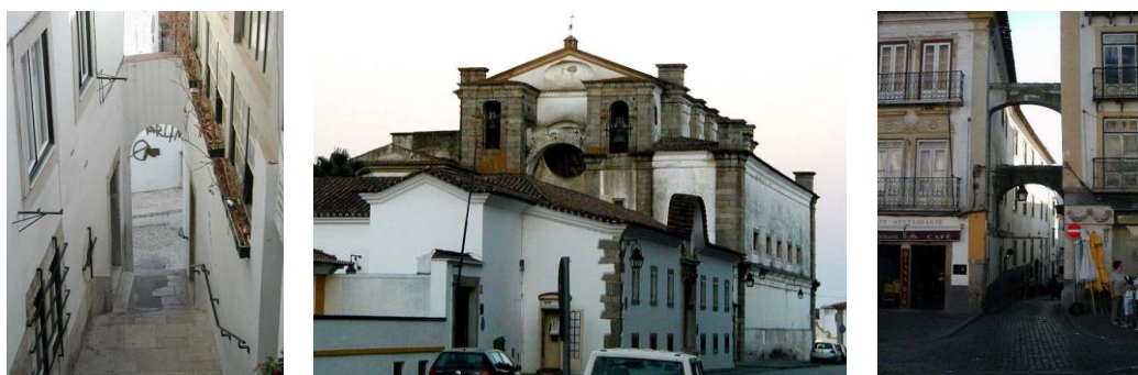
Figure 10. (10a-left) Counter arch in Lisbon, Portugal [12]; (10b-middle) Counter arch in front of the rose window in Igreja do Espírito Santo, Évora, Portugal [12]; (10c-right) Counter arches in Évora, Portugal [12]
