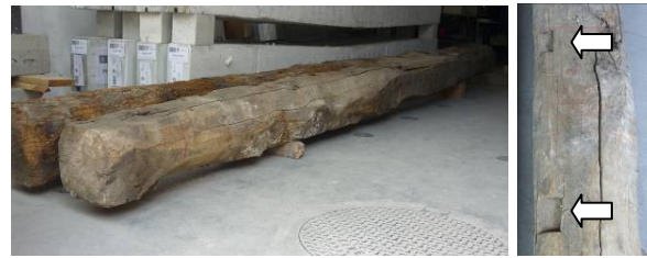
Figure 2: Tested beams with detail of the traditional indentations for the floor support
