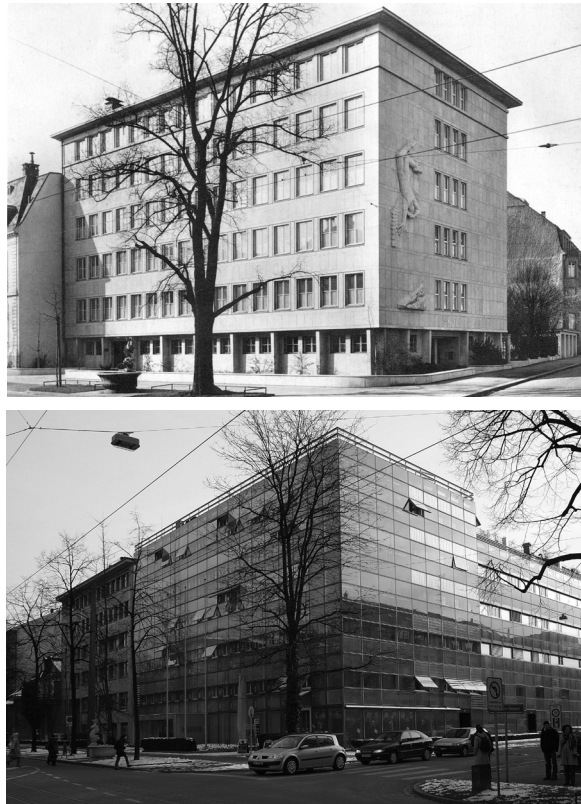
FIG.2 & 3 SUVA building before and after the intervention of Herzog & de Meuron, Basel, 1991-1993.
