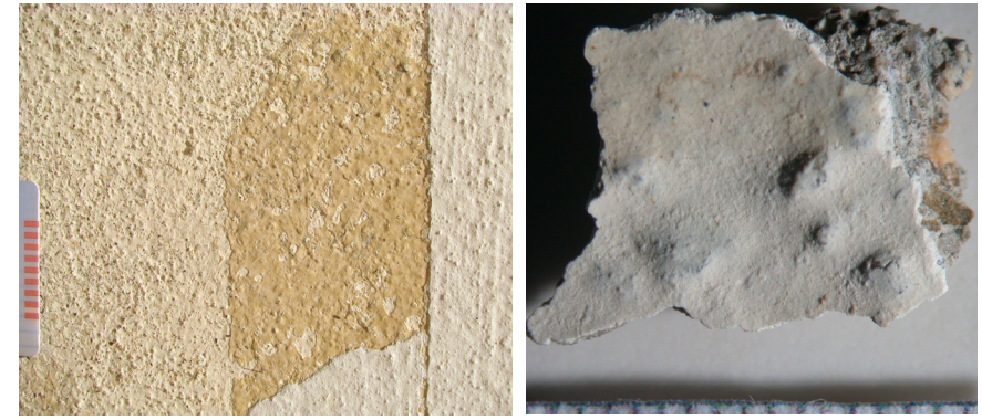
FIG. 15 Upper terrace, façade, detail. The image width corresponds to about 15 cm. Sample of removal of superimposing layers of yellowish limewashes (which were executed before about 1965) and the cement / resin slurry dating from 1985. The stripe on the left: the original surface with the grated plaster with yellowish-white limewash, which is pigmented with fine sand. Photo by Ivo Hammer, 2011.
