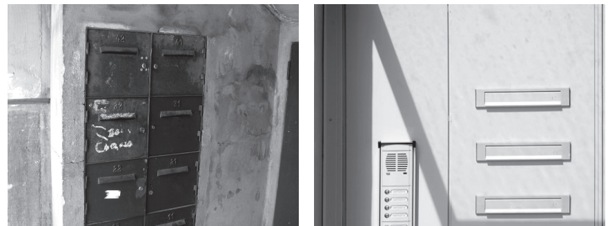
14 The insulation was made under the bays; Regeneration of concrete and rehabilitation of exposed brick / 15 Close off the stairway enclosure, guaranteeing the ventilation in the upper module / 16 Protection of the front door against rain / 17 Ensure old features and create new infrastructures
