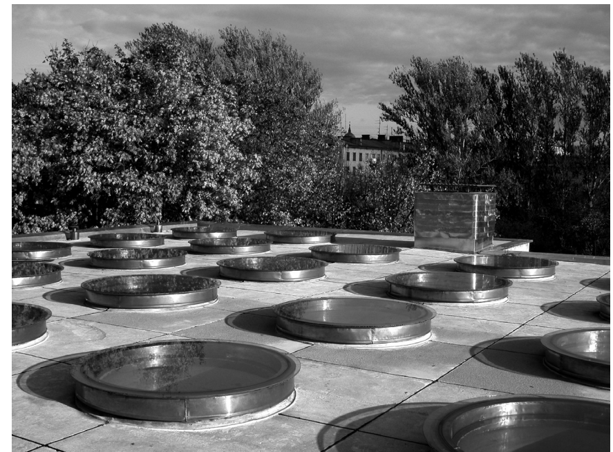
FIG.3 The restored skylights. Photo by The Finnish Committee for the Restoration of Viipuri Library, Maija Kairamo, 2006.
