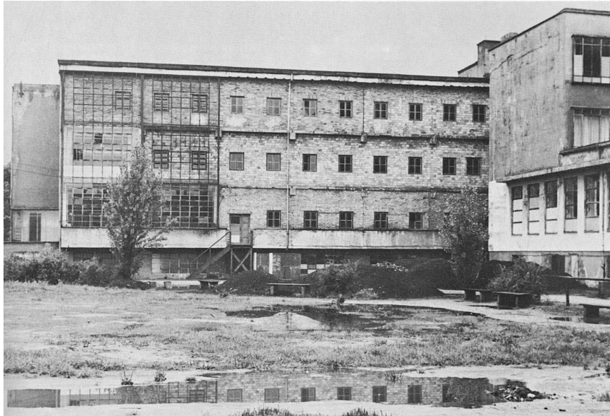
FIG. 1 Bauhaus in ruins photographed by Benevolo in 1956. Pictures like this reinforced the conviction that modern buildings' expendability should be accepted as matter of fact.
