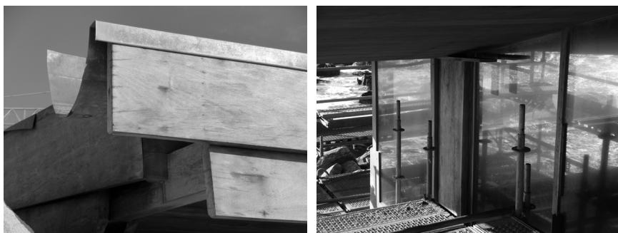
FIG.9 – 10 Casa de Chá da Boa Nova during conservation intervention, 2014. Photos by Teresa Ferreira.
