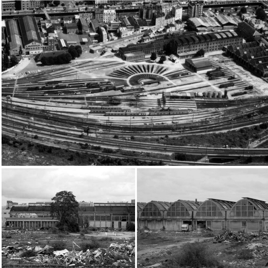
FIG. 3 View of the railway structure.
