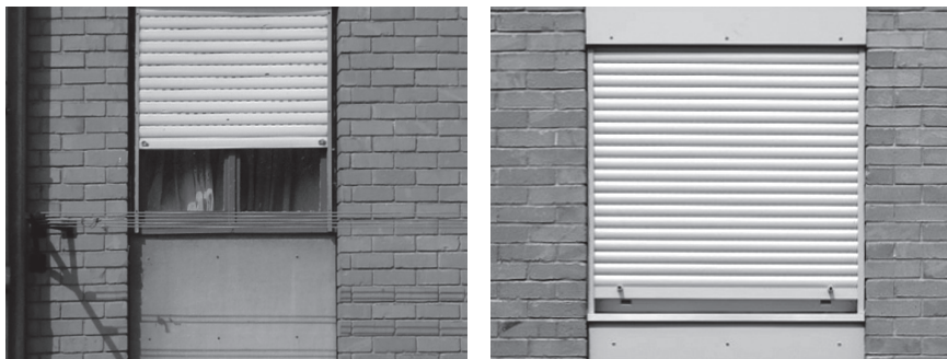
10 Main façade with the new stair case conception / 11 The laundry rooms become a confined space / 12 Laundry rooms - functionality and aesthetics / 13 Placement of double glazing and new frames - a contribution to the thermal and hygrothermal comfort
