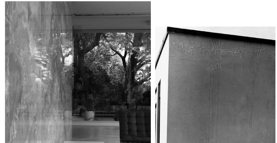
FIG. 9 Main living room, detail of the wall of onyx marble. In the reflection of the architecture and the plants small deviations are shown, which are indicative of the manufacturing process. Photo Ivo Hammer 2012, detail. FIG. 10 Detail of the east façade of the bedroom of Grete Tugendhat. Shortly after the building was completed, cracking of the plaster took place at the intersection of the concrete ceiling and the brick wall caused by different thermal movements of the materials, a built-in drawback created by the combining innovative and traditional techniques. Photo by Rudolf de Sandalo, detail, with original retouche, about 1931
