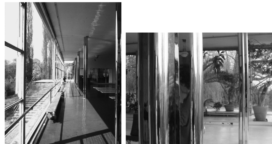
FIG. 7 Main living room when in use as an orthopedic therapy room for the children’s hospital. The only remaining window pane of polished plate glass was very flat, irregularities were hardly noticeable even in the oblique view. The glass panel was allegedly destroyed in the wake of the renewal in 1985. Photo courtesy of Mogens S. Koch, Copenhagen, 1972.
