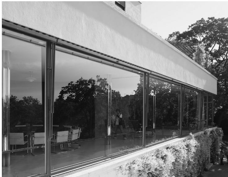
FIG. 20 View from the west, garden facade after restoration. Photo by Jon Soung Kimm, 2012.
