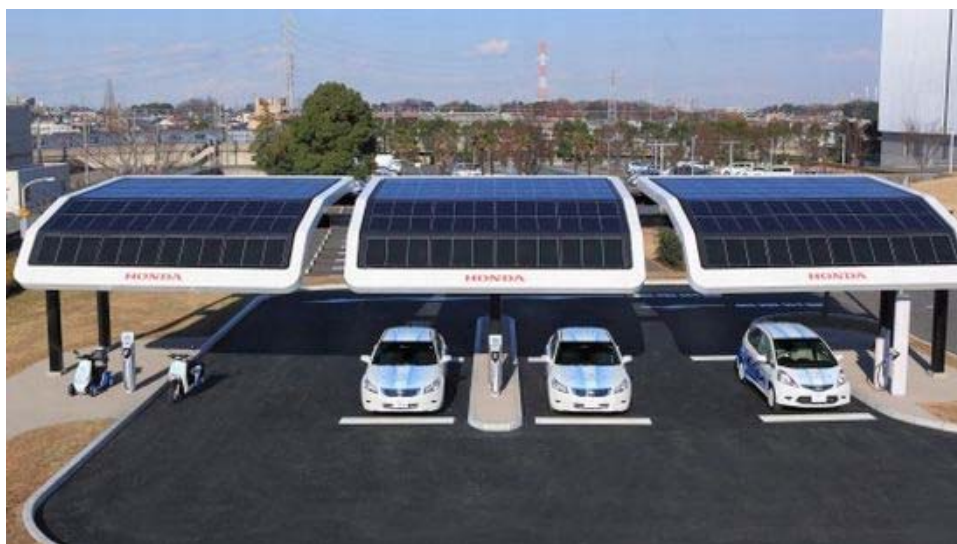
Figure 3-6: Image of a Public charging infrastructure (source from www.ekomiko.pl ). Available charging spots could be a problem since fast charging takes time (more less 10 to 30 minutes (it depends applied power and desirable SOC level))
