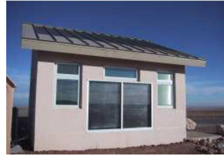
Figura 3.31 Wind Site Entrance Building (SEB) (Colorado, USA).
