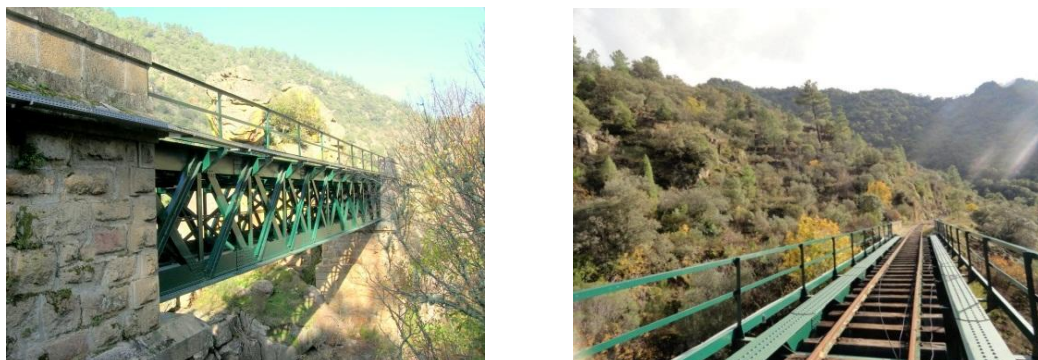
Figure 1 The Paradela Bridge [2]
