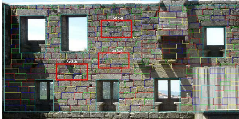
Figure 3: Location of 3x3 Representative Volume Elements (RVEs)
