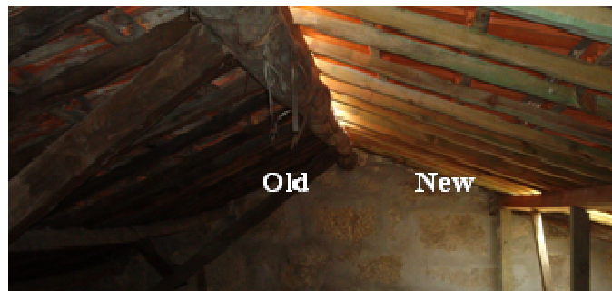
Figure 9. Coexistent old and new timber structural elements.
