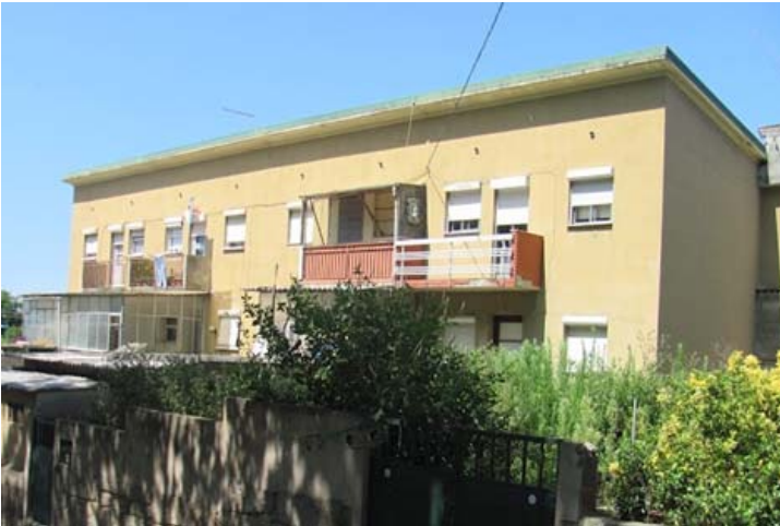
Figure 1: Building before renovation
