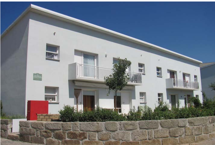
Figure 2: Building after renovation (Base scenario)
