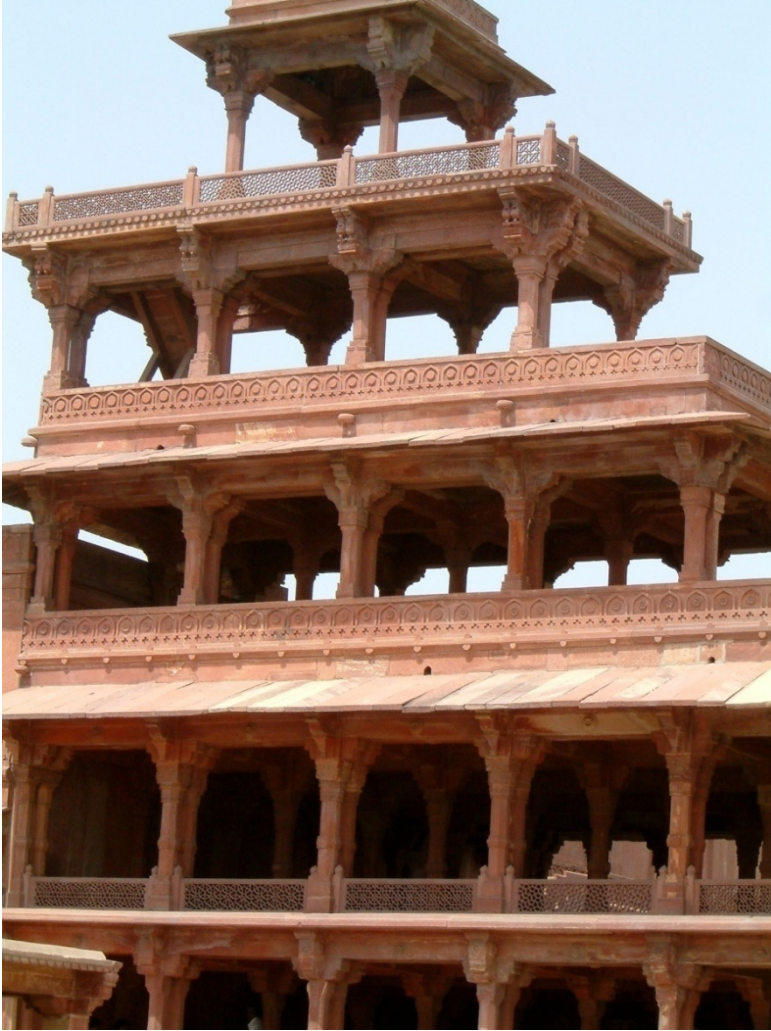
Figure 4. Fatehpur Sikrit, India, built in 16 th century as post-and-lintel construction, obviously inspired by timber construction arrangement and details.
