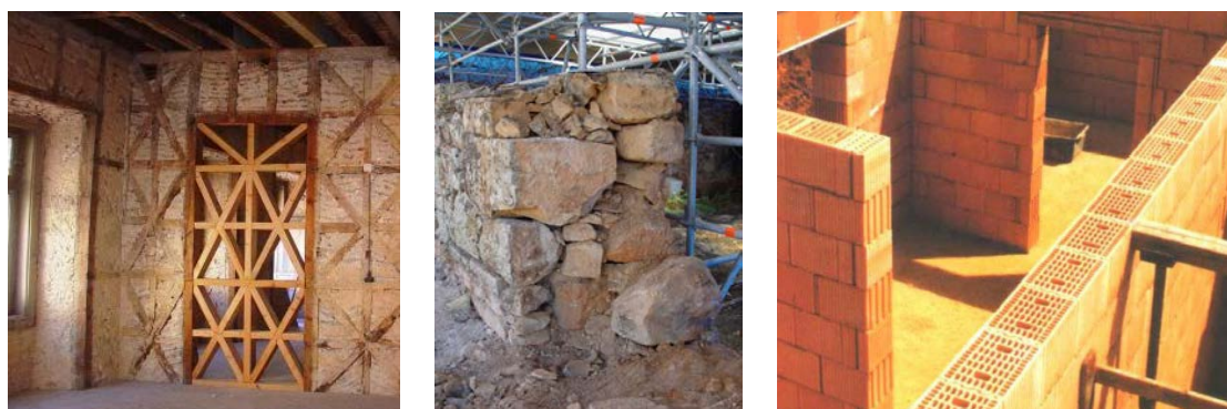
Figure 1. Examples of different masonry types (from left to right): timber braced “Pombalino” system emerging after the 1755 earthquake in Lisbon; irregular stone wall with a complex transverse cross section; unreinforced masonry used in areas of low seismicity using blocks complying with thermal and sound regulations.
