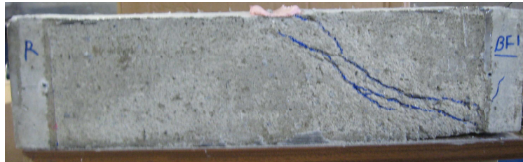
Figure 7: Observation of inclined cracks in BF1 (CFRP was peeled off after the test)
