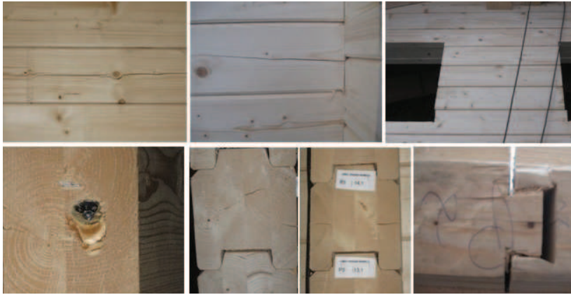
Figure 11. Damages observed in the building after the 0.5g PGA test
