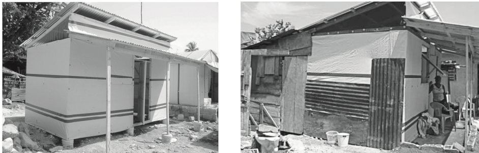
Figure 1. Housing unit before being used and after the user modifies it. The modifications increased the vulnerability of the construction. ( http://openarchitecturenetwork.org ).
