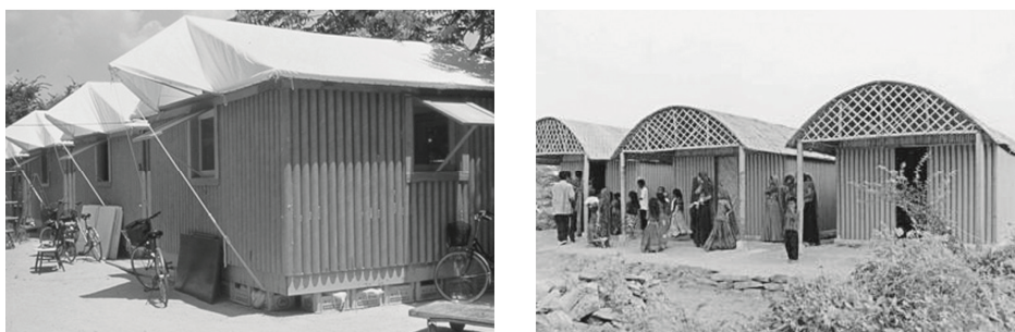
Figure 3. Paper Log Houses: (left) solution used in Japan and (right) the solution used in India ( http://www.shigerubanarchitects.com/ ).
