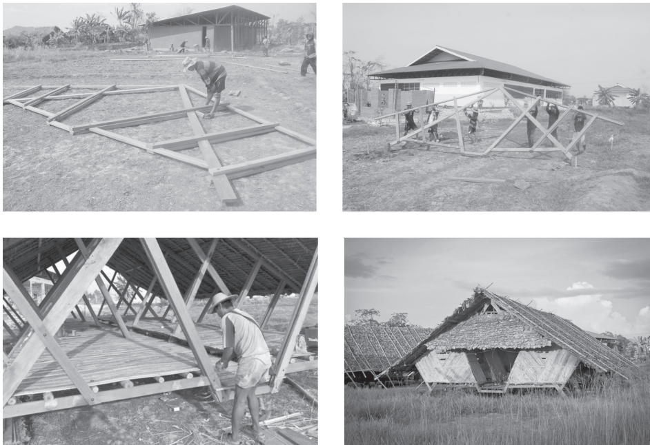
Figure 2. A simple and safe structure built with materials locally available and erected only with manpower through traditional construction. The assembly and maintenance is easy because the construction techniques and materials are well known for users ( www.openarchitecturenetwork.org ).
