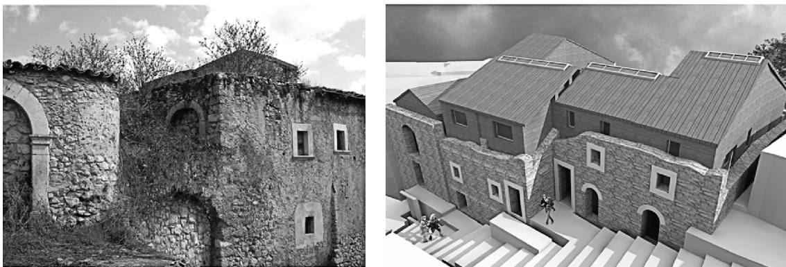
Figure 2. Existing buildings and proposal with the insertion of the wooden volumes (Forlani et al. , 2012).
