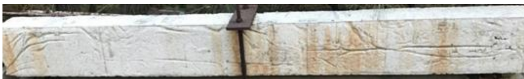
a) GFRP RC beam B3-G-60m
